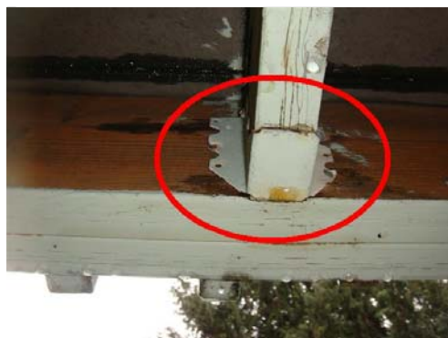
1.1 Item 2(Picture) Example of fasteners needed
