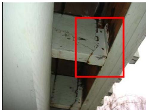
1.1 Item 3(Picture) Example of fasteners needed
