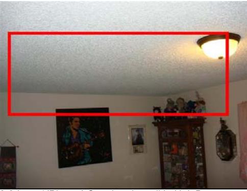
8.2 Item 1(Picture) Sagging drywall in Unit B
