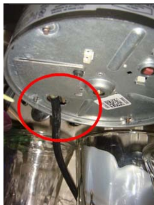
10.6.B Item 1(Picture) Connector needed
