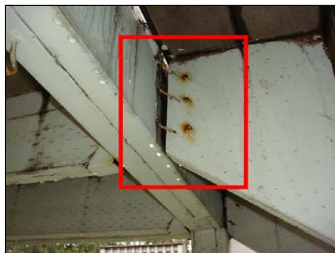
1.1 Item 5(Picture) Stair stringer pulling loose
