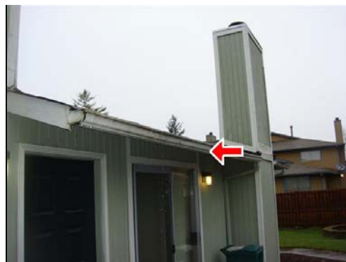
4.3 Item 2(Picture) Water overshooting the gutter
