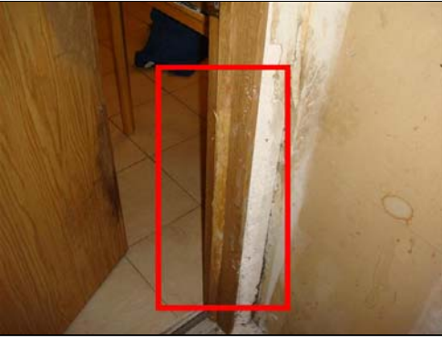
9.3 Item 1(Picture) Damaged jamb in Unit C
