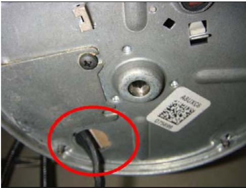
10.6.D Item 1(Picture) Connector needed
