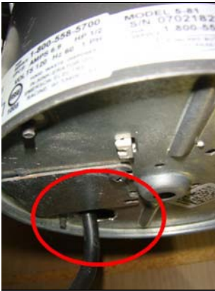
10.6.C Item 1(Picture) Connector needed
