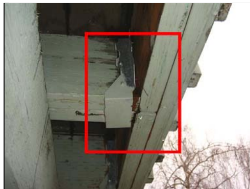
1.1 Item 11(Picture) Example of fasteners needed
