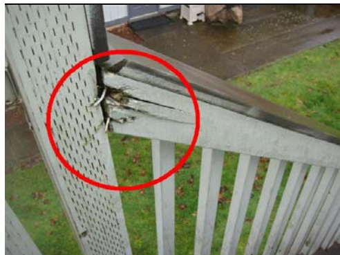
1.1 Item 16(Picture) Damaged handrail
