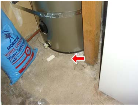
5.2 Item 6(Picture) Thermal barrier needed in Unit A
