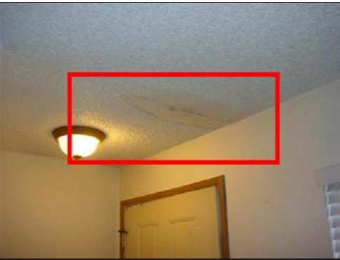
8.2 Item 3(Picture) Evidence of prior leak in Unit C
