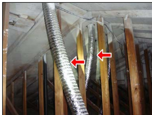
4.6 Item 2(Picture) Non-insulated ducts
