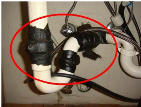
10.1.C Item 2(Picture) Nonprofessional repairs
