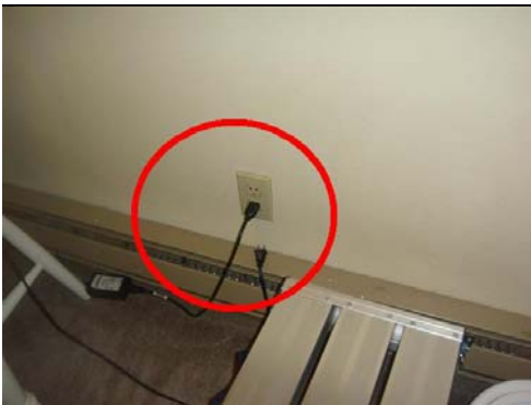
7.3 Item 1(Picture) Example of outlet above the baseboard heat
