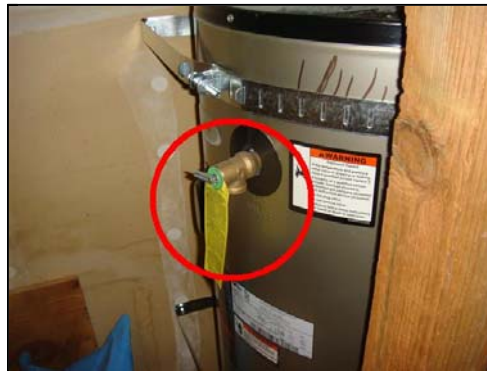
5.2 Item 4(Picture) No discharge pipe on Unit A
