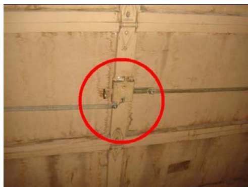
9.2 Item 2(Picture) Handle missing Unit C
