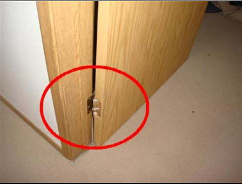
8.5 Item 1(Picture) Disconnected hinge in Unit C
