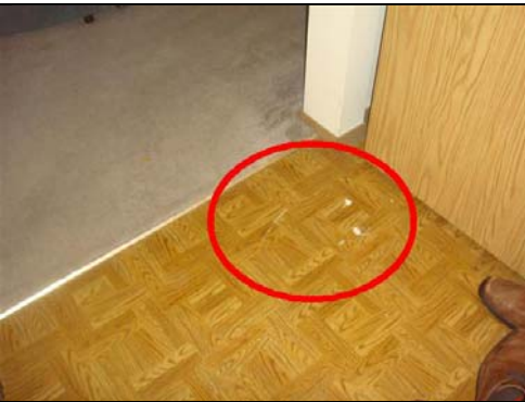
8.4 Item 1(Picture) Damaged vinyl flooring in Unit A
