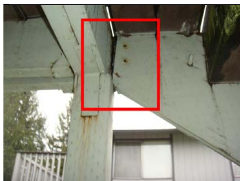
1.1 Item 6(Picture) Stair stringer pulling loose
