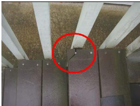
1.1 Item 15(Picture) Example of cracked composite stair treads
