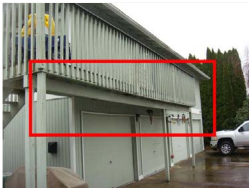
1.1 Item 10(Picture) Location needed fasteners
