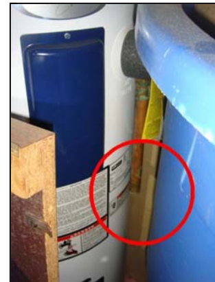
5.2 Item 5(Picture) Discharge too short in Unit D
