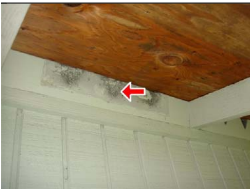
4.5 Item 1(Picture) Minimal ventilation
