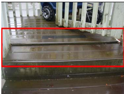
1.1 Item 12(Picture) Evidence of settling where stairs meet deck
