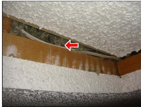
7.2 Item 4(Picture) Electrical subject to damage
