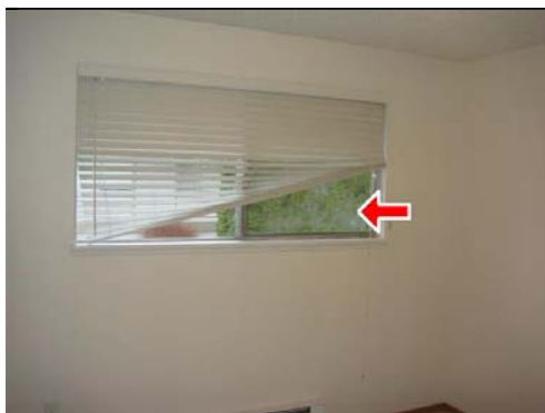
8.7 Item 3(Picture) Failed thermal seal unit C
