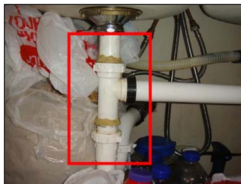
10.1.D Item 2(Picture) Nonprofessional repairs
