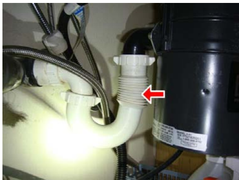
10.1.C Item 1(Picture) Ribbed drain
