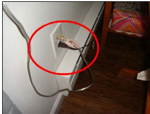
7.3 Item 2(Picture) Example of outlet above baseboard heat
