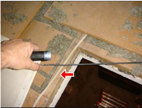
7.2 Item 3(Picture) Electrical subject to damage
