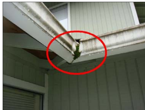
4.3 Item 5(Picture) Example of leaking gutter
