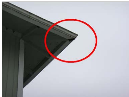
4.3 Item 3(Picture) Example of leaking gutter
