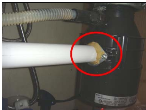
10.1.D Item 1(Picture) Nonprofessional repairs
