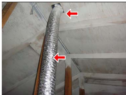
4.6 Item 1(Picture) Duct tape/non-insulated duct
