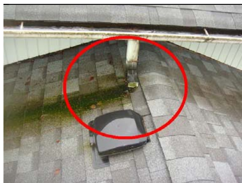
4.3 Item 8(Picture) Poor downspout termination
