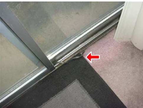
8.6 Item 1(Picture) Damaged weather seal Unit A
