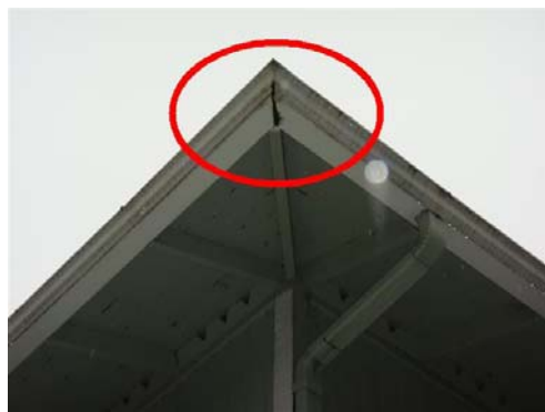
4.3 Item 1(Picture) Example of leaking gutter
