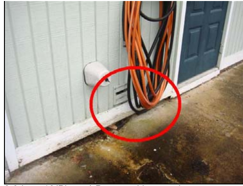
2.0 Item 18(Picture) Damaged louvered cover
